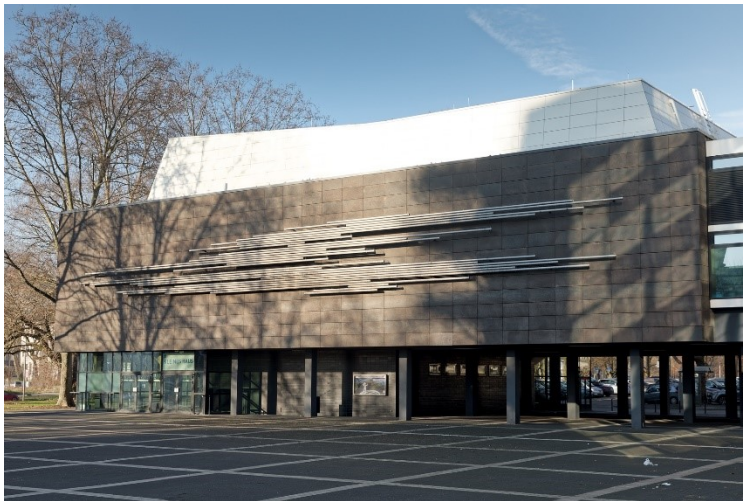
The south wall of the “Kleines Haus” is decorated with a relief of metal pipes created by the sculptor Norbert Kricke
